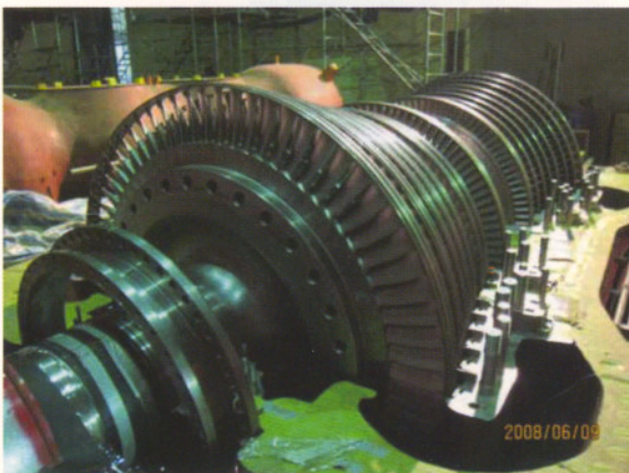
圖1. 1號機高壓汽機安裝作業
